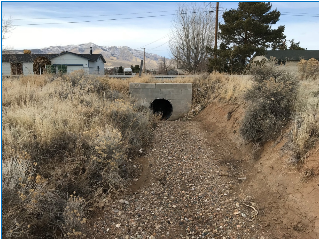
Existing culvert at Estates Road into which the channel drains.
